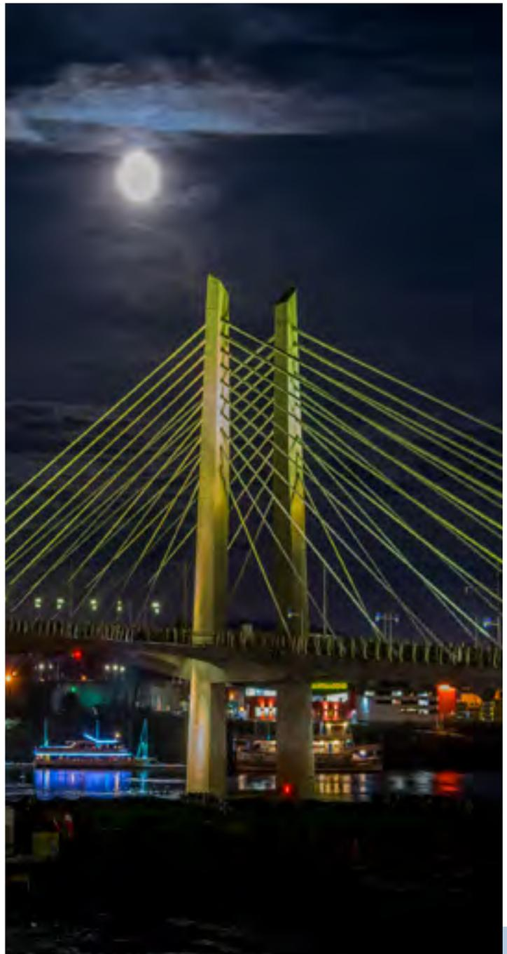
*The river's speed, height and temperature is translated into real-time aesthetic lighting for Tilikum Crossing, using 178 LED light bulbs.*
